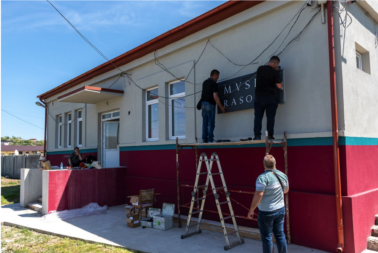
Installing the panel for the Museum Rasova
