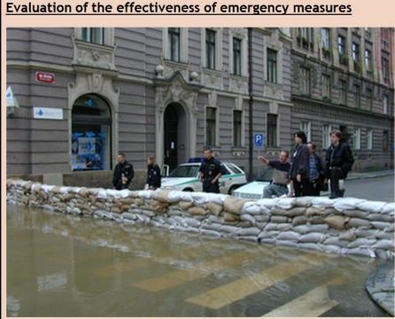
Some emergency measures provide a relatively fast and cost effective protection against floods. However, their effectiveness can be limited and it should be always taken into consideration for each measure the safe uses that are allowed. For example, the employment of sand bags is successfully applicable only at low depth and slow velocity of water flow.
