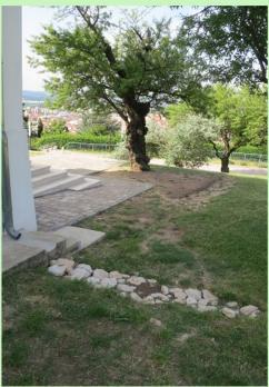
Existing drainage systems should be surveyed and repaired on a periodic basis. New systems, or parts of them, should be carefully designed to allow for the increased rain loads. in case the existing system is deemed not sufficient. In this example, drain pits have been added to the system in order to stop the flowing of water downhill (notice the erosion of the ground due to rain before interventions).
