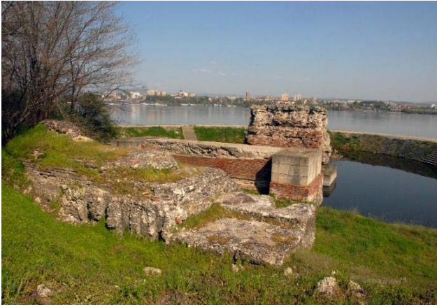
Fig. 3.5.5. Pons Traiani / Trajan's Bridge between Kostol (Pontes) and Drobeta (Romania). Piers on the Serbian bank of Danube – present day situation (© Nemanja Mrđić, Archive of the Institute of Archaeology).
