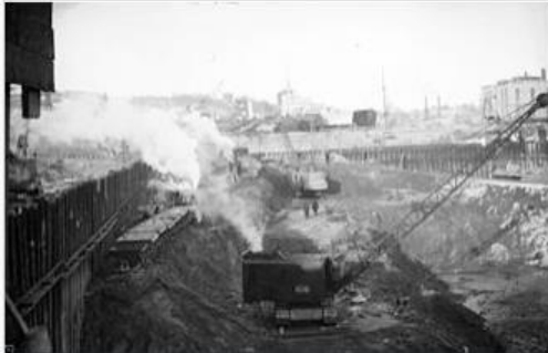
Construction of the bunker
