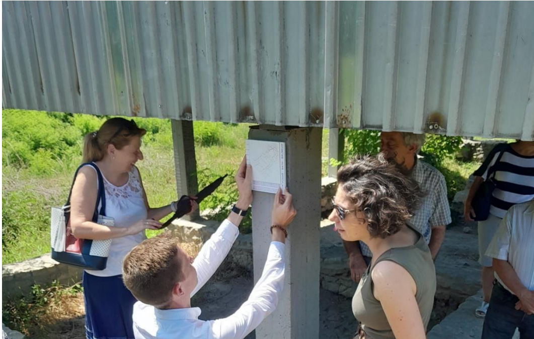
Fig 9: Installation of the VR Board on the Pilot Site – the traces of the Roman Bath of Matrica, Százhalombatta, Hungary. (see D.T.2.3.2: Implementation of virtual reality reconstructions on pilot sites).
