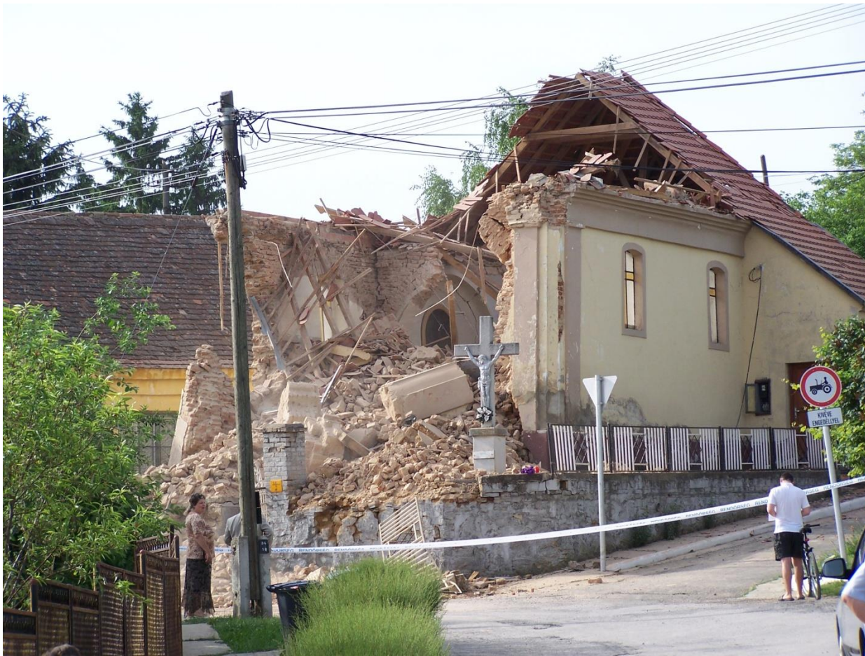
Collapse of the Roman Catholic church of Belyárdgyula, 2006
