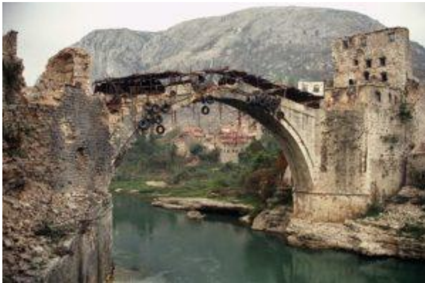
Demolition of the bridge of Mostar, 1993
