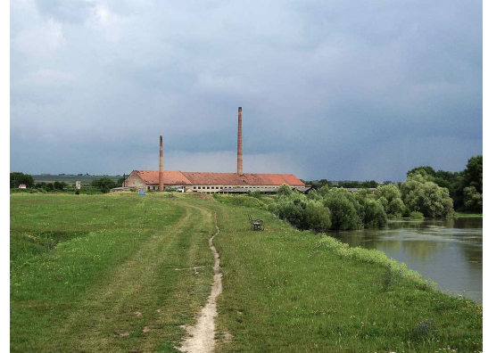
Figure 13: A possible site of the Roman fort Teutoburgium
